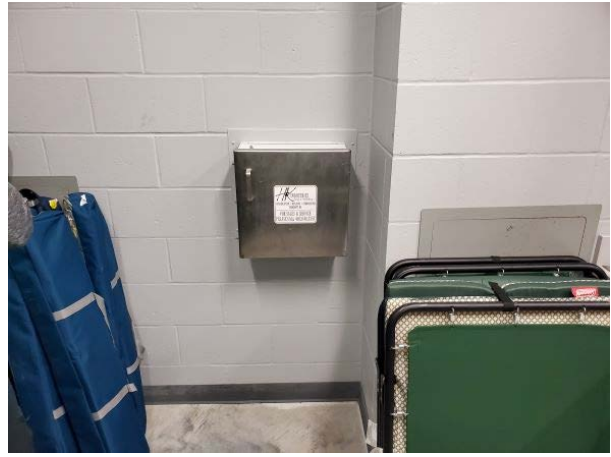
Figure #2. Welded clothing transfer between Storage and Intake Shower Room
