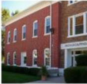
EXISTING COURTHOUSE & PONCA
