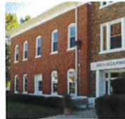
EXISTING COURTHOUSE & PONCA
